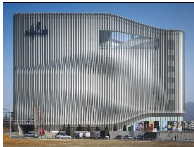
Figura 6: Galería Center City – UNStudio – Fuente: https://www.unstudio.com/en/page/388/galleria-centercity
